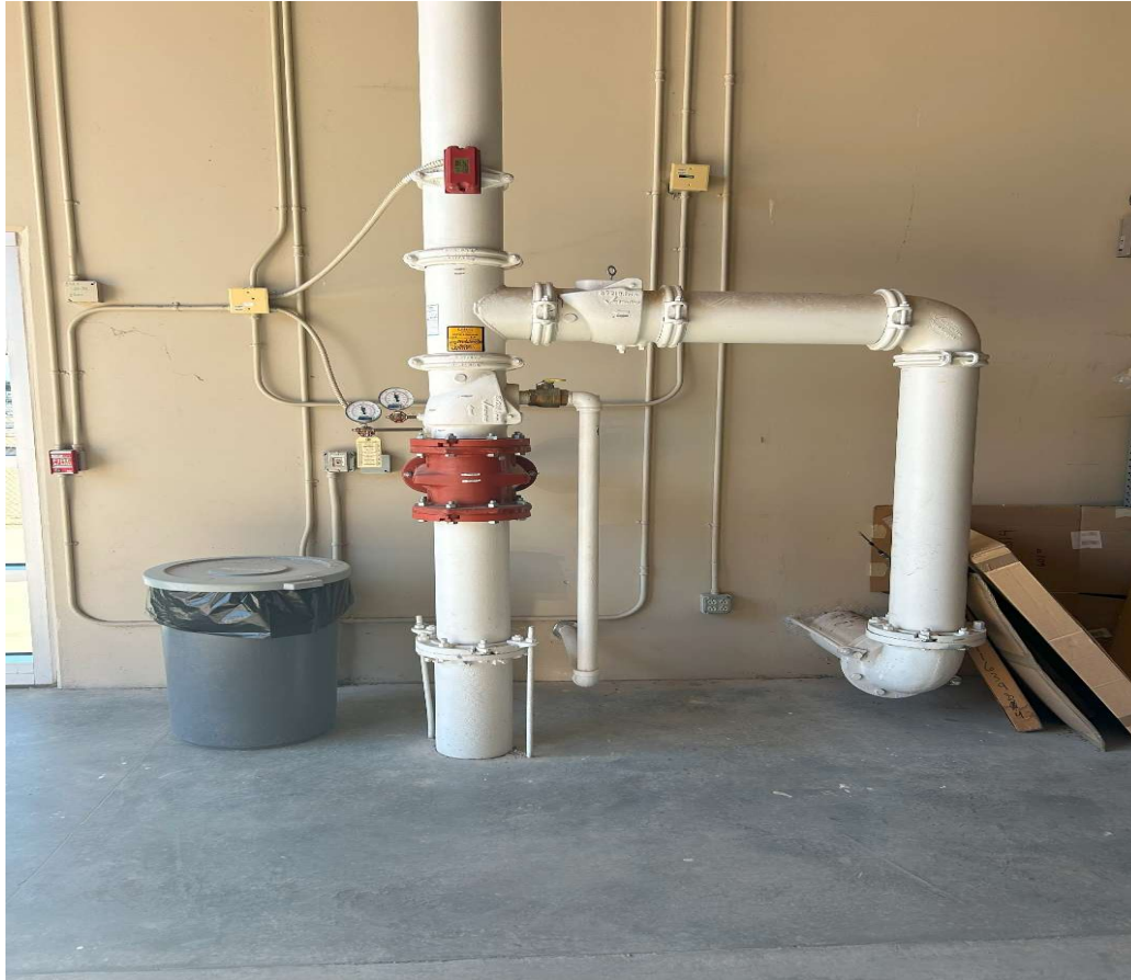
Fire riser in storage warehouse
