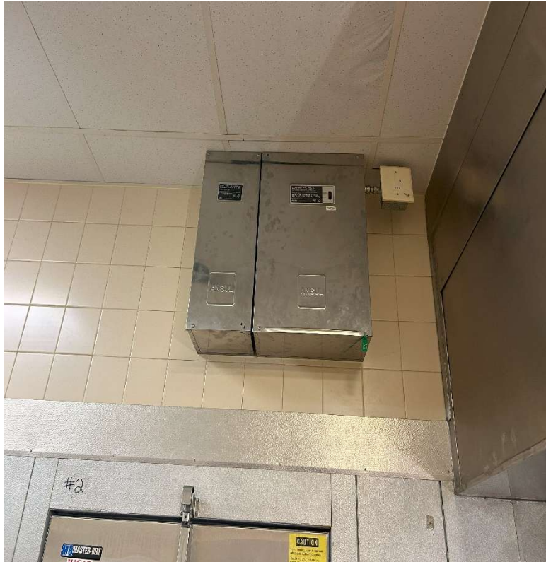
Kitchen Suppression system. 3 tanks serving 2 hoods
