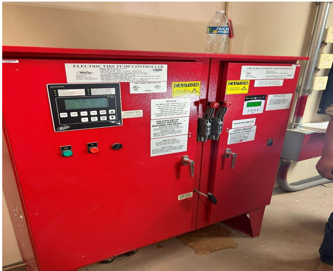
Fire pump controller
